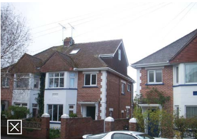
Fig 5.19: Unacceptable as the side dormer alters the symmetry of the pair and harms the original design integrity of the existing building
