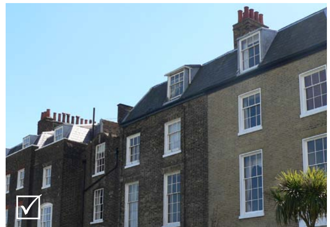
Fig 5.11: Acceptable due to its slender, subordinate form and alignment with the elevation below
