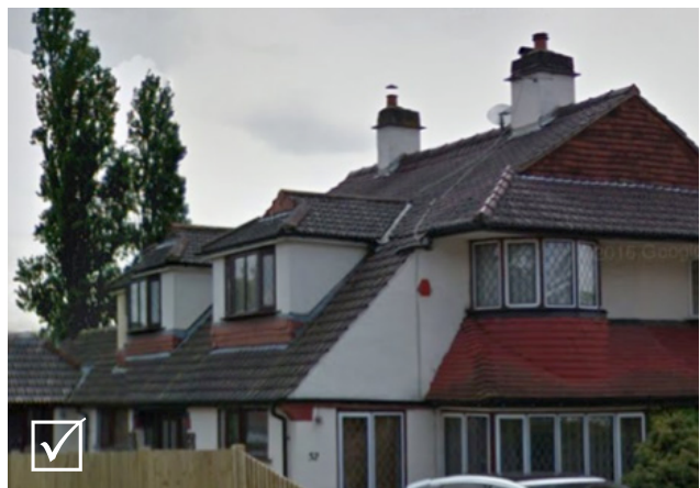
Fig 5.20: Acceptable as the side dormers are subordinate to the roof and set in from all directions
