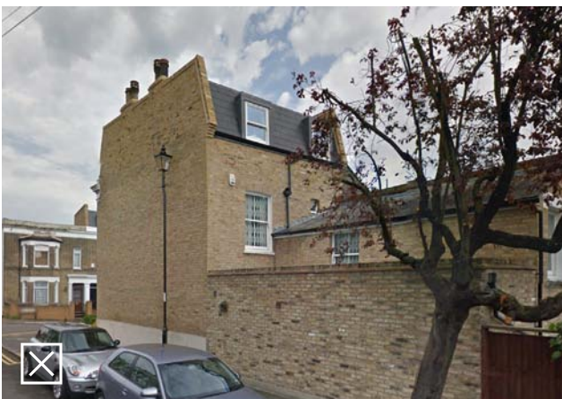
Fig 5.35: Unacceptable - Roof extension does not retain butterfly roof form
