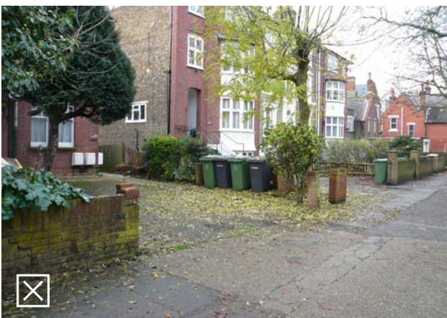
Fig 6.5: Unacceptable due to its harmful impact to the street scene
