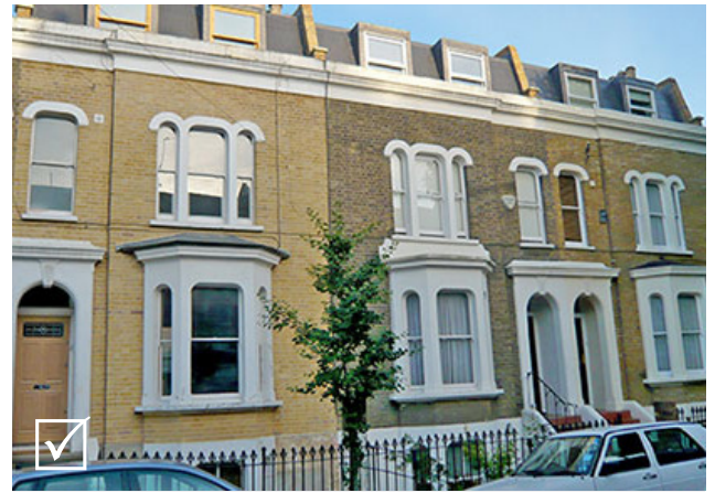
Fig 5.33: Acceptable example of mansard roof extension from the front behind existing parapet. All extensions are similar dimensions and look uniform
